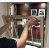
Step 2 - Using the D handle or ring pull slide the sash back up to the top of the frame.
