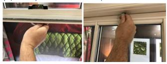
Step 2 - Slide up the bottom sash using the lift hooks. The sash can only go as far up as the sash stops on either side to keep the sash level.
