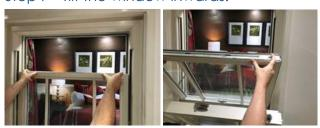
Step 4 - Once the bottom sash is tilted you can tilt in the top sash.
